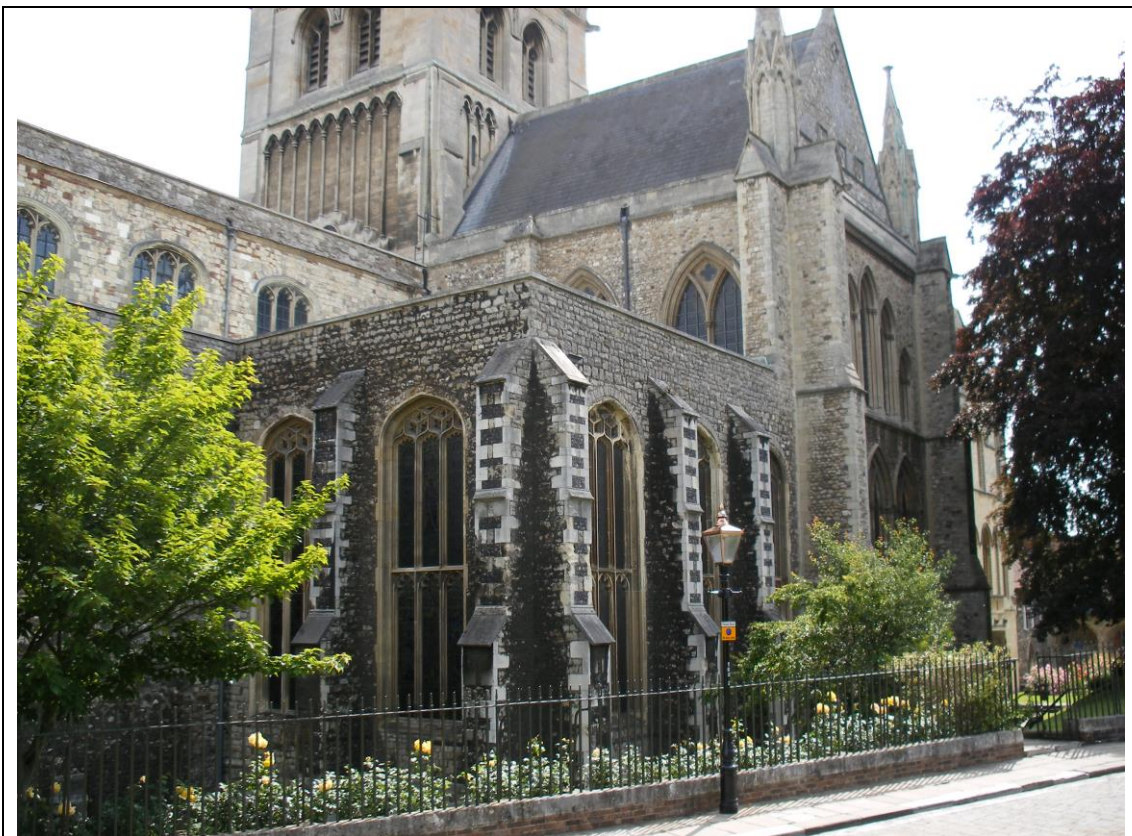
The Lady Chapel (foreground) and South Transept seen from the west.
