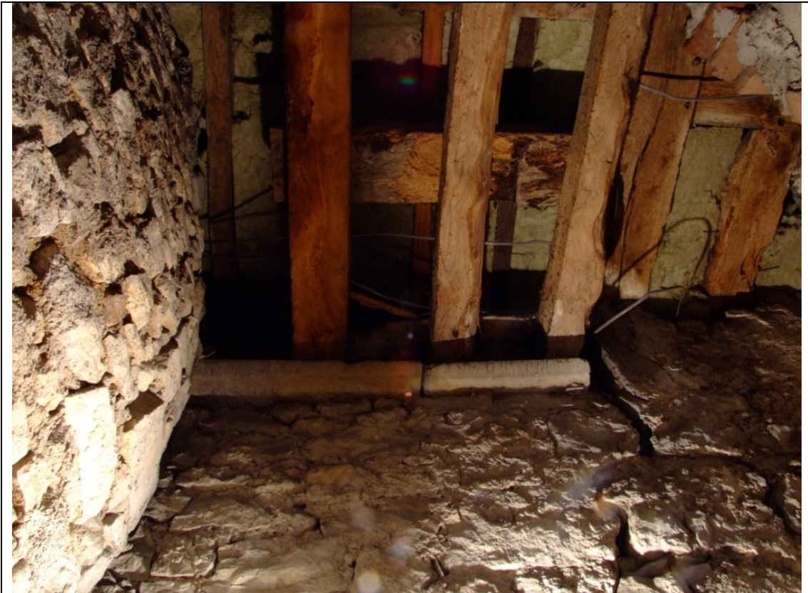
Figure 14: The west wall (3) of Deanery Gate, with the cill and jamb of a window, re-used as the seating for floor joists. Note the structural crack running down from the jamb.
