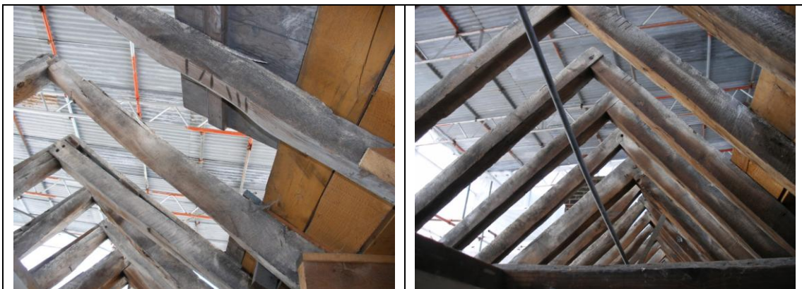
Figure 9: The west roof seen from the east (left) with the IIIIII tally on the underside, and from the west with the II-III tallies on the side. The timbers marked IIIIII and IIII are the same pair.
