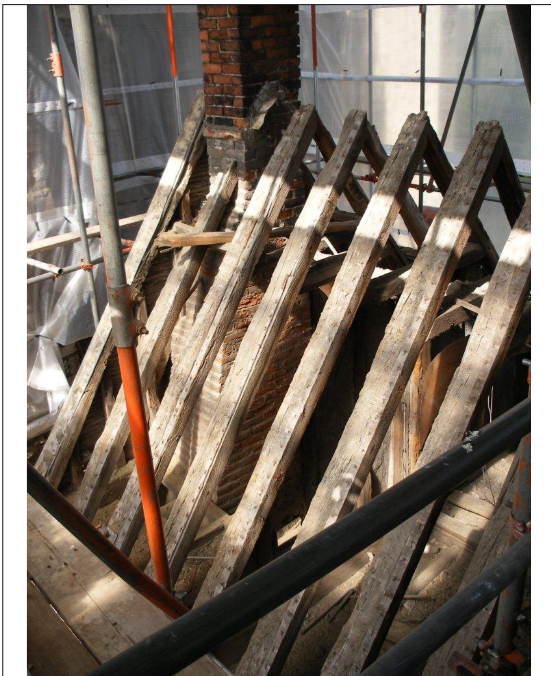
Figure 1: The roof over the Deanery Gate during repair works in July 2007.
