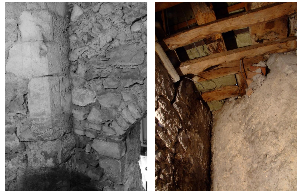
Figure 13: The polygonal turret, with the cross-wall abutting it (left) and the front wall of the Deanery Gate cutting across it (right). The window cill can just be seen towards the top left of the right-hand photograph.
