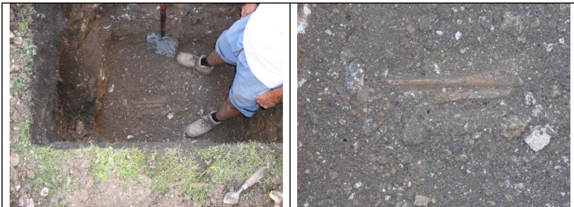
Figure 5: The foundation pit during excavation showing the human bone in grave 4. Note the brick rubble in the left-hand photograph.
