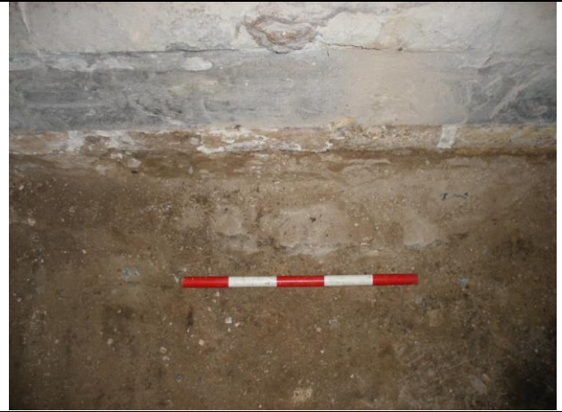
Figure 6: Detail of offset foundation 1006.
