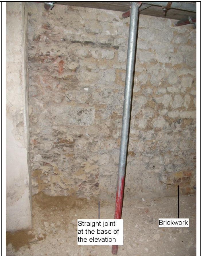
Figure 5: The same bay in March 2010 with the failed render removed to reveal the masonry behind it. Note the straight joint, highlighted.
