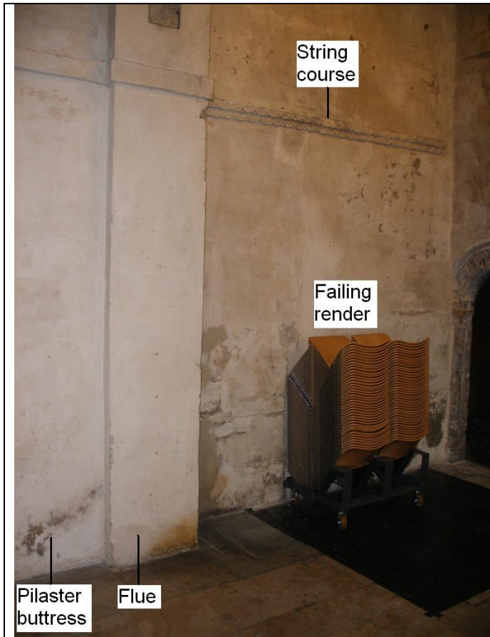
Figure 4: The westernmost bay of the south aisle in October 2009, before work started. Note the string course.
