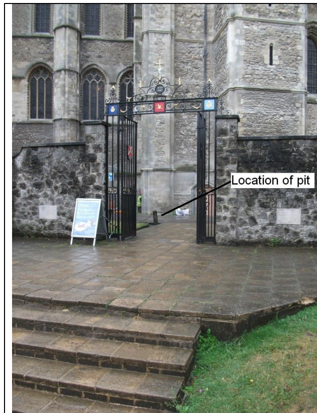
Figure 2: Location of the foundation pit seen through the gates from the Memorial Garden, with the Cathedral's east end in the background.
