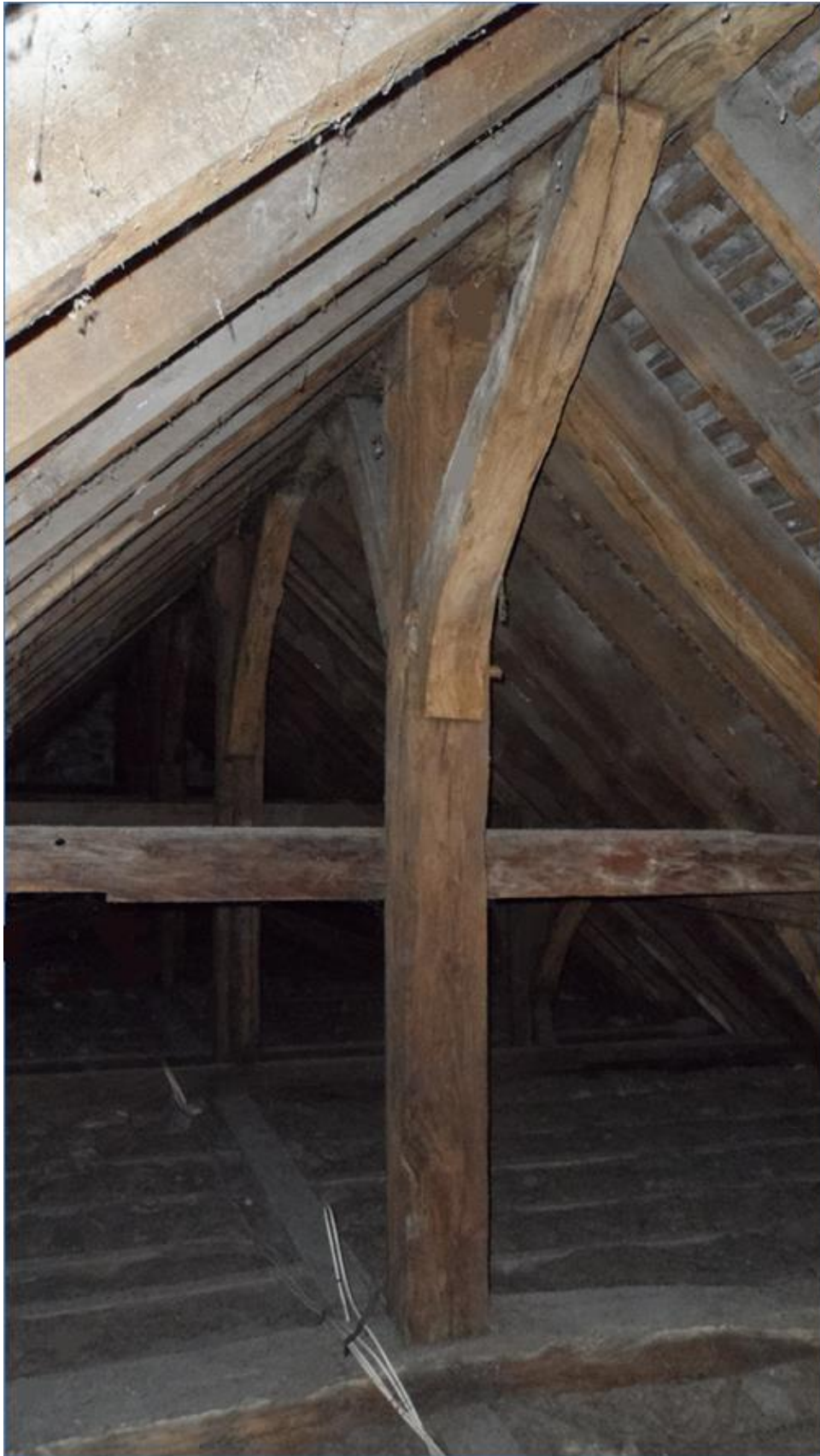
Figure 5: Chapter Room roof, truss 6 in foreground
