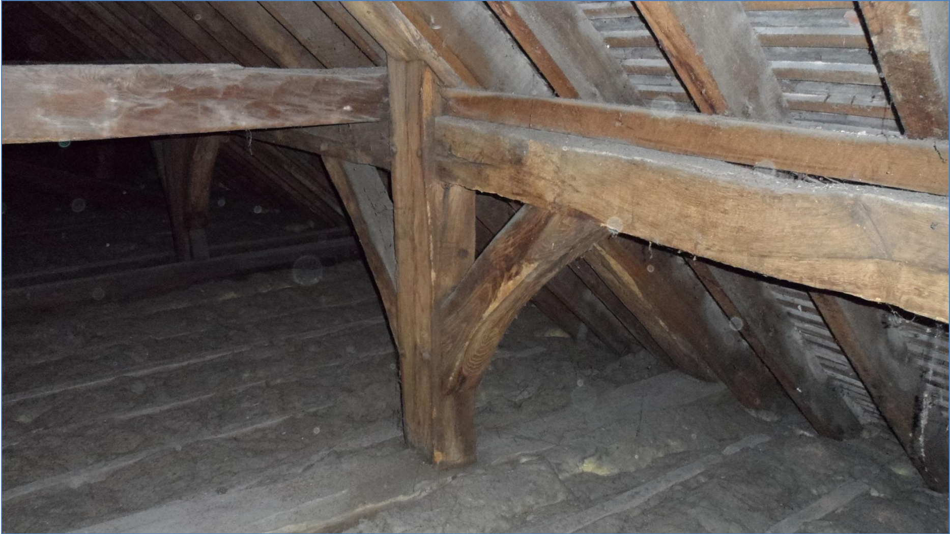
Figure 6: Chapter Room roof, south side
