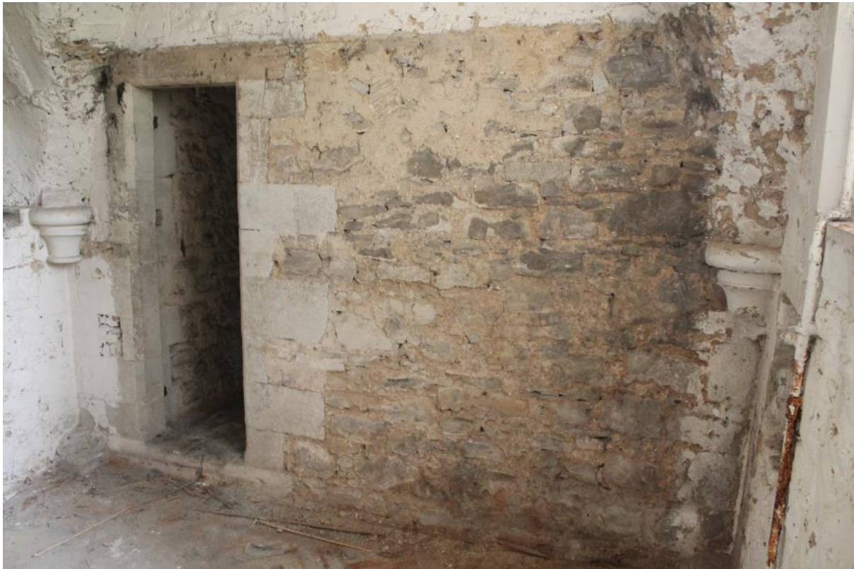
Plate 29: The east wall of the side-crypt (former cleaner's store) cleared of shelving in August 2014. The door to the mural passage and (blocked) stairs and the remnants of the engaged colonette shafts were exposed as expected.
