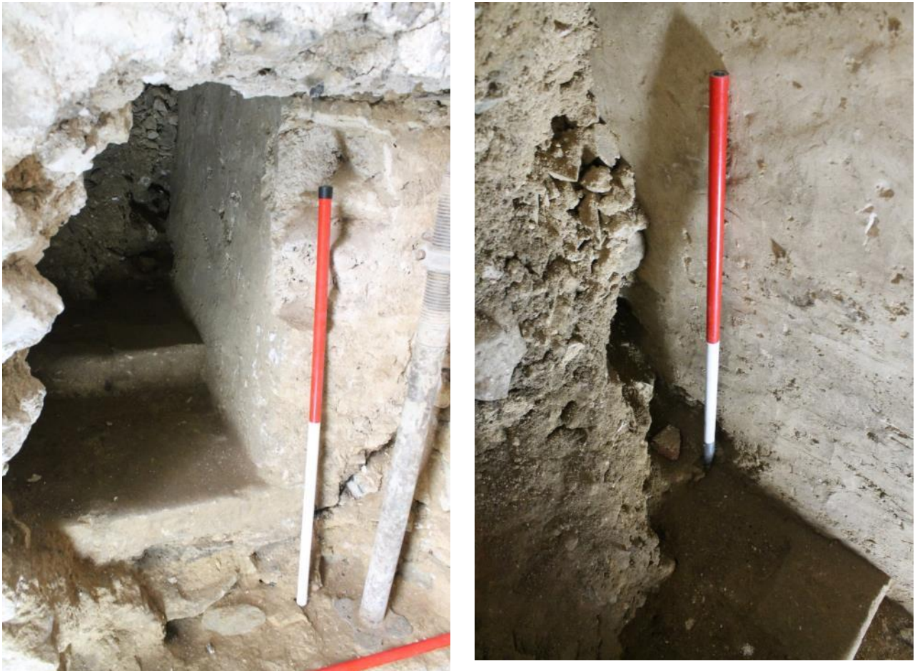
Plate 31: The north jamb (with its tufa blocks), threshold and step exposed behind the west wall of the store. The 'ghosts' of two further steps are visible in the right-hand photograph. Scale 1m in 0.5m sections.
