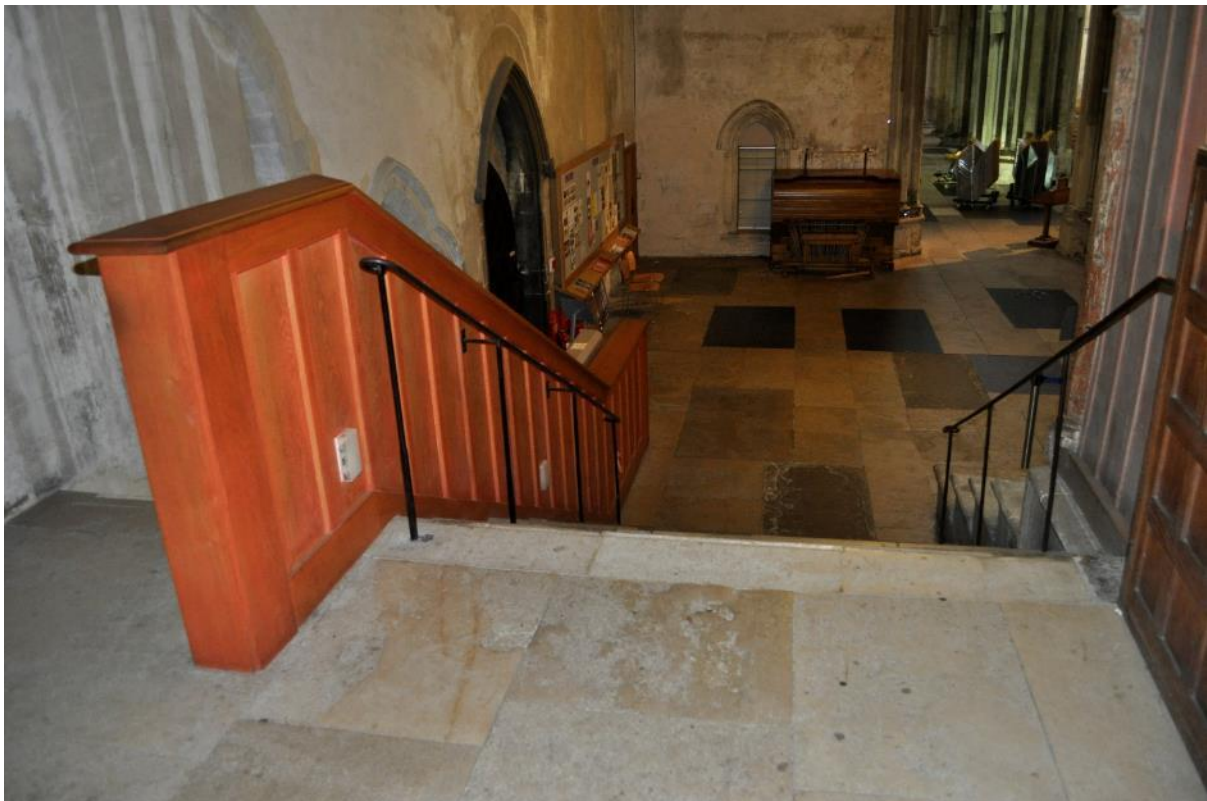
Plate 3: The South Quire Aisle and the Kent Steps looking east in 2014, before the main contract began, showing the change in floor levels. The timber structure to the left hid the wheelchair lift.
