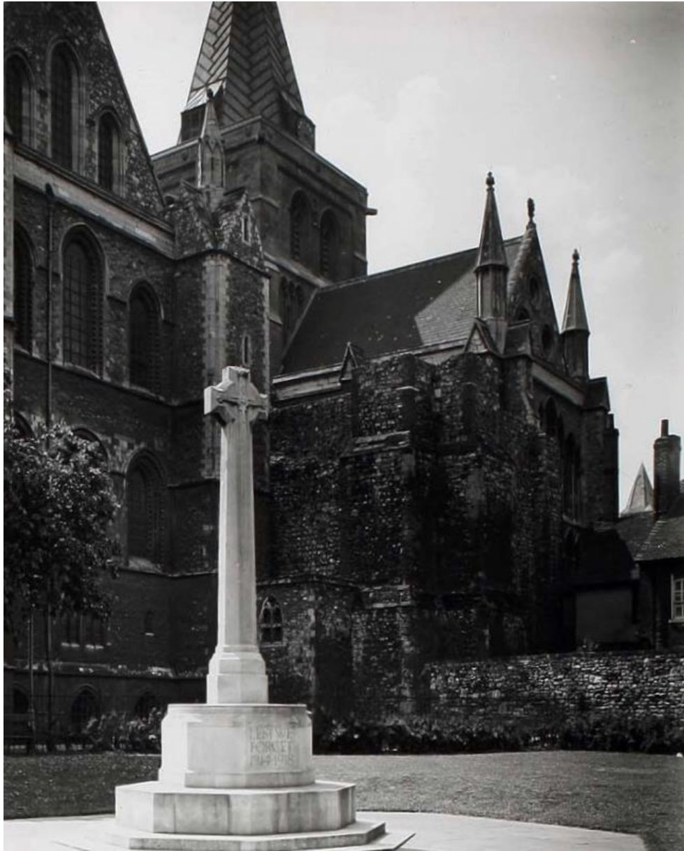
Plate 7: Gundulf's Tower with its massive clamping buttresses, to the right of the War Memorial, in 1936. Historic England Archive image AA52/5142.
