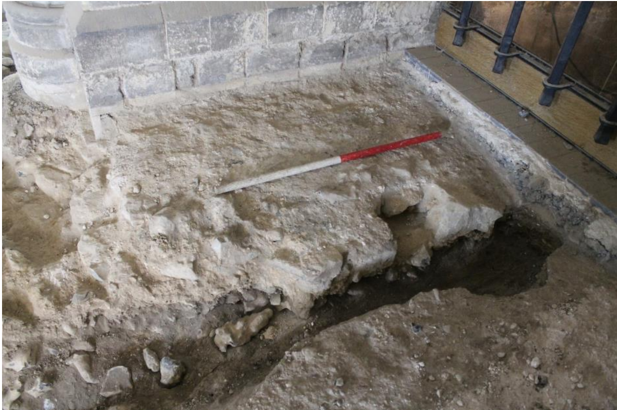
Plate 22: The south face of wall 724, with the dressed blocks showing that this was originally standing fabric. The foundations can be seen where one stone had been removed in antiquity. One of the late 12 th -century piers at the entrance to the Ithamar Chapel had been built directly onto the Norman wall, though a small area of new footing was needed on its north side.
