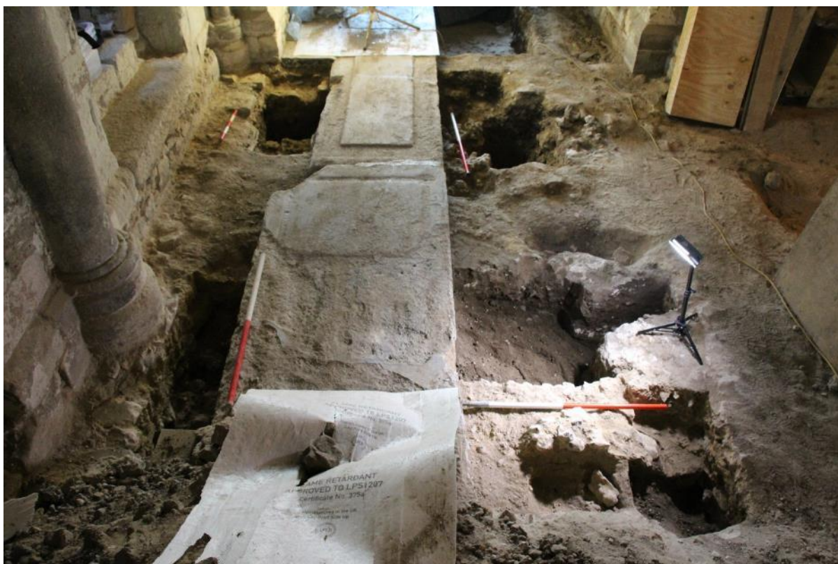
Plate 25: Walls 840 (in the foreground) and 842 (under the rear right scale), with the path of re-set ledger stones separating them. The north foundation of the Norman crypt is to the right, thickened at the east end (ie the north-east corner), perhaps to support a pilaster buttress. View looking east.
