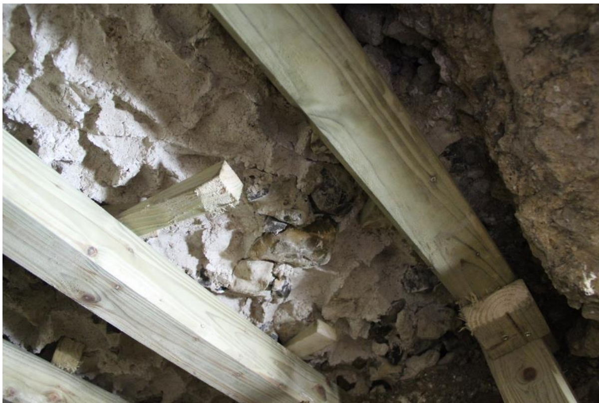
Plate 28: Mortar and flint floor 1221 formed the roof of Irvine's tunnel. The rough underside of the poured surface is very evident here. The small hole referred to in the following paragraph can be seen starting to open up to the right of the trench shore closest to the crypt wall.
