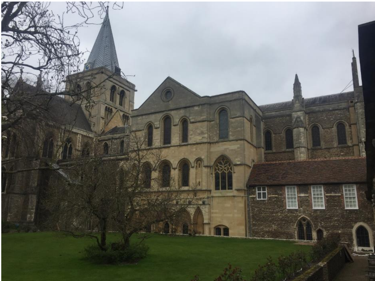
Plate 2: The cloister and eastern arm of Rochester Cathedral looking north-west. The two-storey building at bottom right is the Chapter Library (on the first floor), with the vestry beneath.
