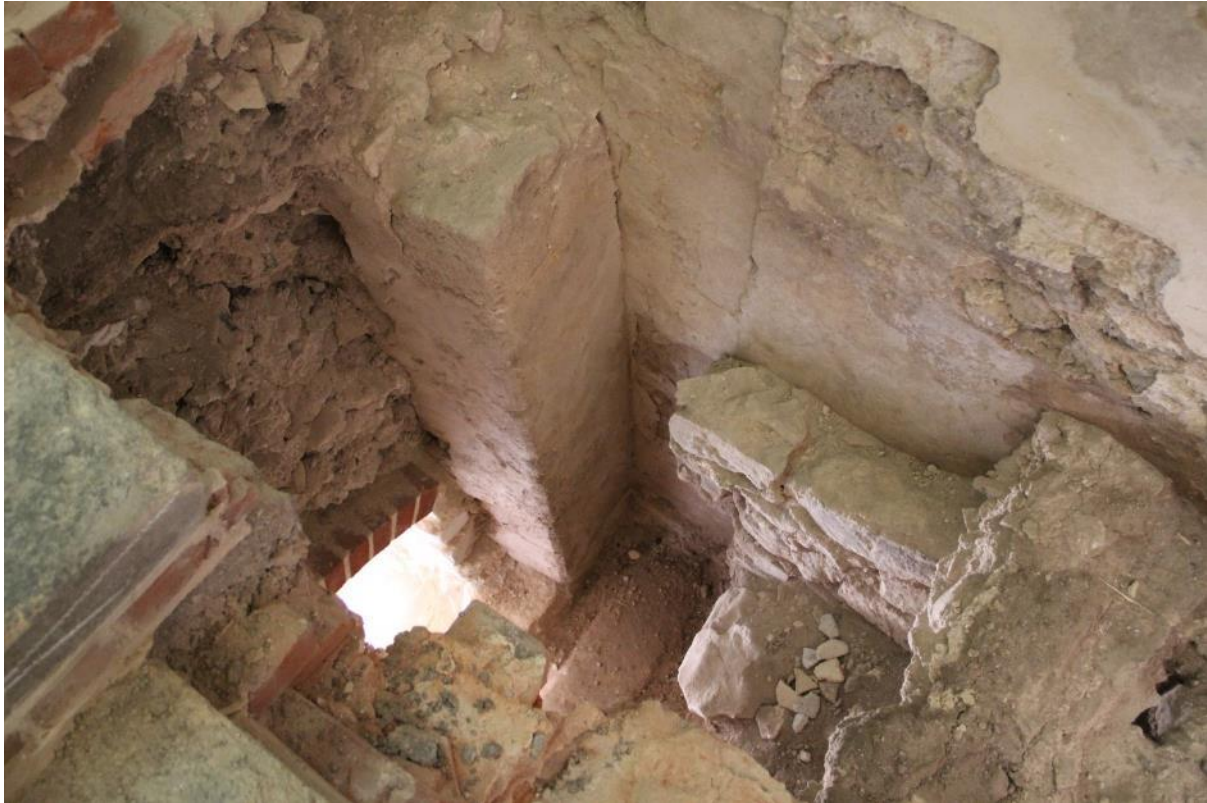
Plate 32: View of the Norman remains in the lift pit excavation, with jamb 214 butting against wall 215. The window jamb to the west of 214 is clearly visible, with infill 213 blocking it. Note the outline of the removed treads of the Kent Steps at top right as well.
