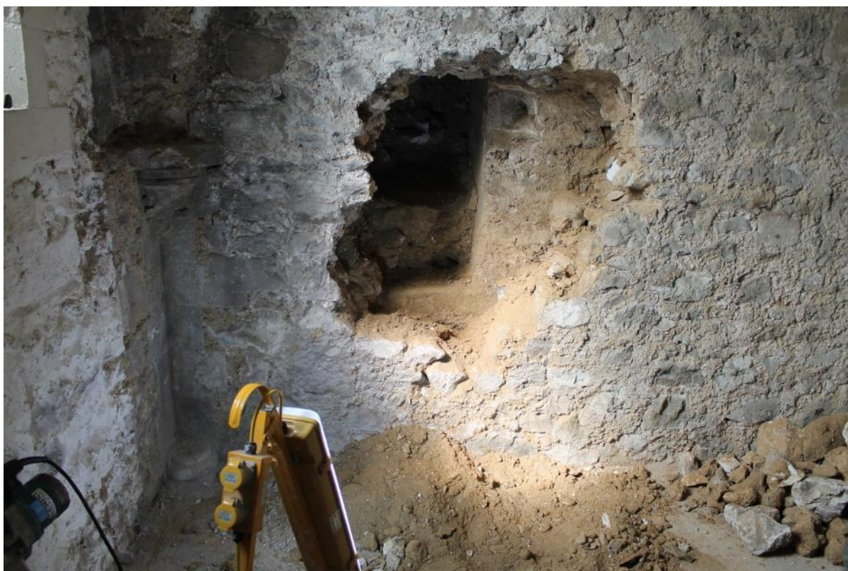
Plate 30: The gradually expanding hole in the west wall of the side crypt on 19 September 2014, a few days after the masonry had first been exposed. It was becoming clear that one side (the jambs) and a threshold step of a doorway had been found, but this had to pre-date the 1179 fire which had caused the rebuilding of the eastern arm and crypt of the Cathedral.
