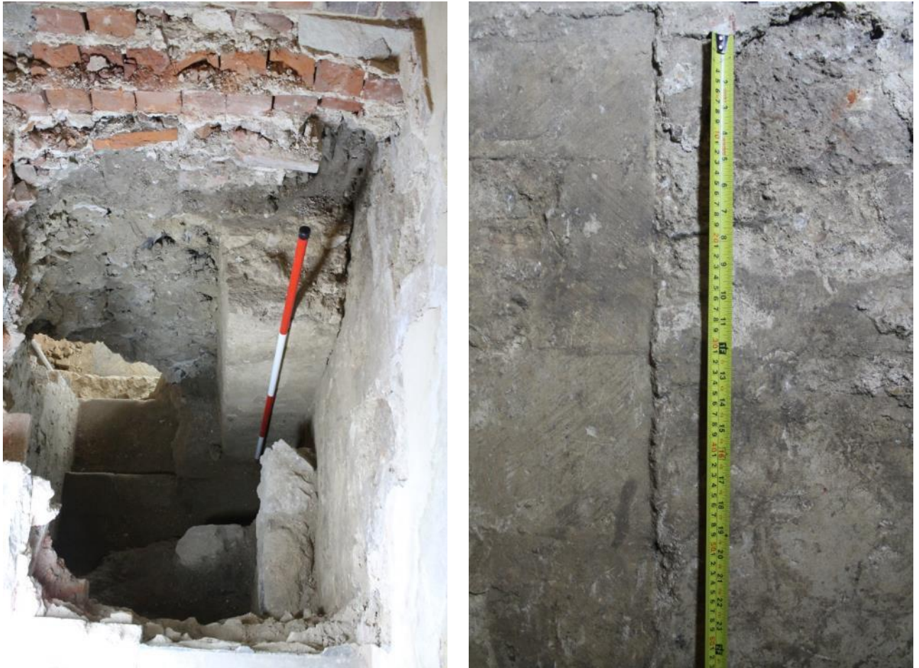
Plate 33: Left – the door jambs seen from behind, ie the west, with the wall of the South Quire Aisle to the right. Scale 2m, in 0.5m sections. Right – the jambs of what must be a window – it does not continue to floor level – with later (presumably late 12 th /early 13 th -century) rendered blocking to the right. Note the high quality and crisp condition of the tooling on the jamb stones.
