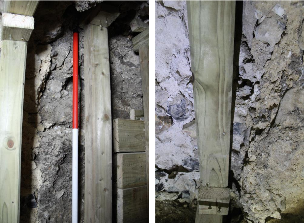
Plate 27: Left – the south face of Irvine’s tunnel re-opened. The dark earth and Roman soils can be seen behind the lower (white) portion of the 1m scale, with the made ground behind the red upper part – the sloping tip lines can be seen to the right. Note the rough rear (west) face of the crypt wall to the left. Right – the north side of the tunnel with mortar and flint floor 1221, and the crypt wall to the right. The shadows cast by the arc light clearly show that the floor both abuts and slightly overlaps with the wall.
