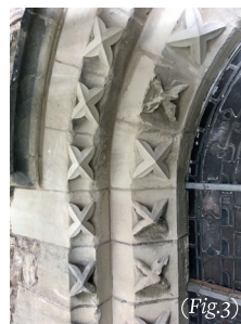
Restored decorative details.
