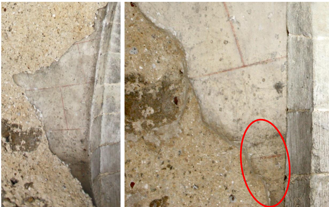
Fig 3. Island of plaster on Area L soffit before and after TAC cleaning. The discoloured lower part is the most suitable for (B) samples. (B) samples (2 x limewash, 2 x paint) = 4 (B) samples.
