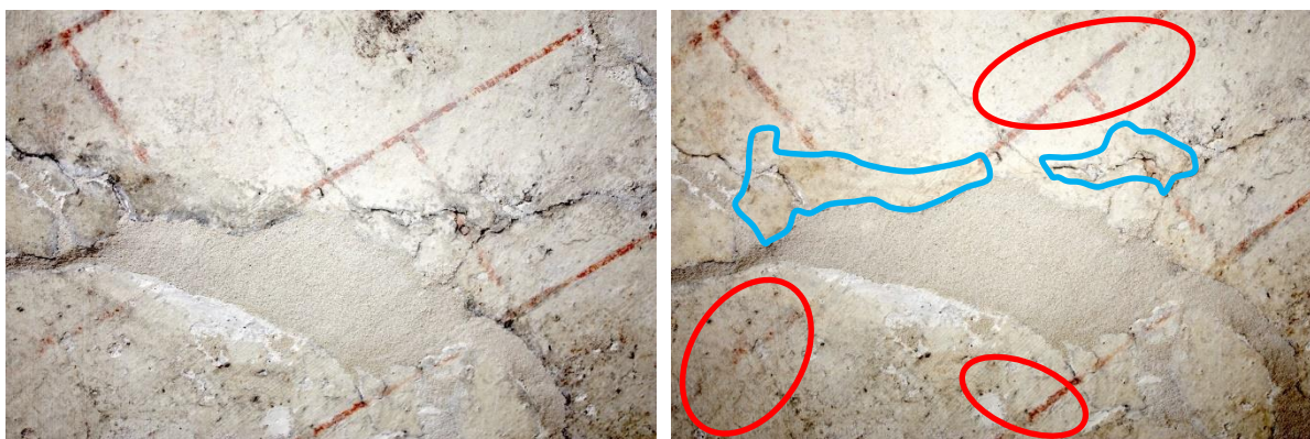
Fig 4. Detail of ingrained dirt along the edges of a crack in the Bay 13c vault plaster, before ( left ) and after ( right ) spot laser cleaning. Areas outlined in red are suitable for B samples but only for comparison with the adjacent (C) sample areas (outlined in blue) since, uniquely, the whole of Bay 13 was overpainted at an early stage with a plain red ochre layer. (B) samples (2 x limewash, 2 x paint) = 4 (B) samples . (C) samples (2 x limewash, 2 x paint) = 4 (C) samples .
