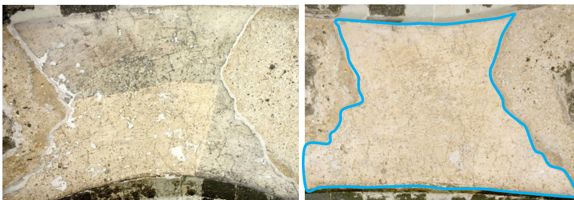
Fig 7. Details of Area K soffit plaster during ( left ) and after laser cleaning ( right ). It is unlikely (B) samples will be obtained from this arch soffit plaster. The area outlined in blue is suitable for (C) samples (2 x limewash, 2 x paint) = 4 (C) samples .
