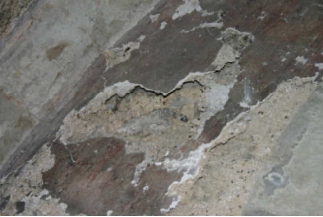
Plates 5&6: Details of the lower central area, showing the severely delaminated section of painted plaster before (above left) and after (above right) treatment.
