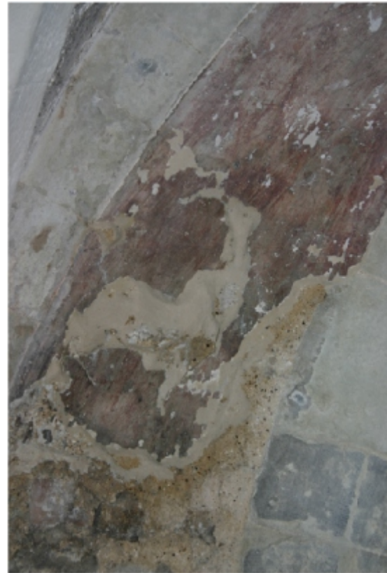
Plates 3&4: Details before (above left) and after (above right) treatment. A plaster bridge was built up consolidate vulnerable edges prior to injection grouting.
