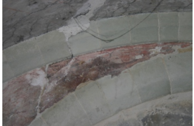
Plates 8&9: Details of the upper area of the spandrel, before (above left) and after (above right) treatment. Plaster fillet repairs were applied to delaminating edges and a grout injected into voids in the area to the right of the vertical crack. The large piece of white, later inappropriate repair plaster was removed, to reveal the original painted surface.
