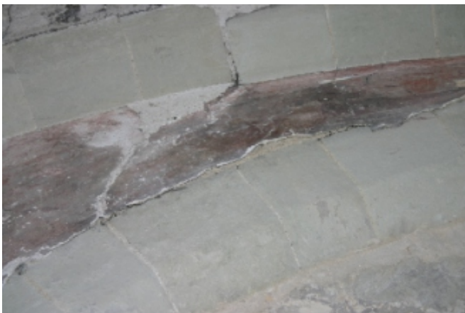
Plates 8&9: Details of the upper area of the spandrel, before (above left) and after (above right) treatment. Plaster fillet repairs were applied to delaminating edges and a grout injected into voids in the area to the right of the vertical crack. The large piece of white, later inappropriate repair plaster was removed, to reveal the original painted surface.
