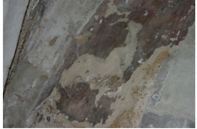
Plates 5&6: Details of the lower central area, showing the severely delaminated section of painted plaster before (above left) and after (above right) treatment.
