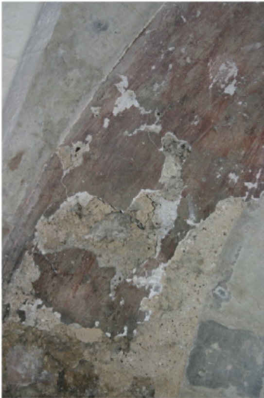
Plates 3&4: Details before (above left) and after (above right) treatment. A plaster bridge was built up consolidate vulnerable edges prior to injection grouting.
