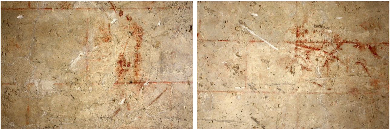
Fig 5. (above) . Area E arch soffit. Raking light details showing scrapes and indents: accidental impact damage which has occurred since the 2013 Phase 1 treatment works.
