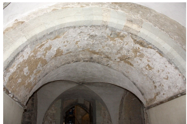
Fig 5. (above) . Area E arch soffit. Raking light details showing scrapes and indents: accidental impact damage which has occurred since the 2013 Phase 1 treatment works.
