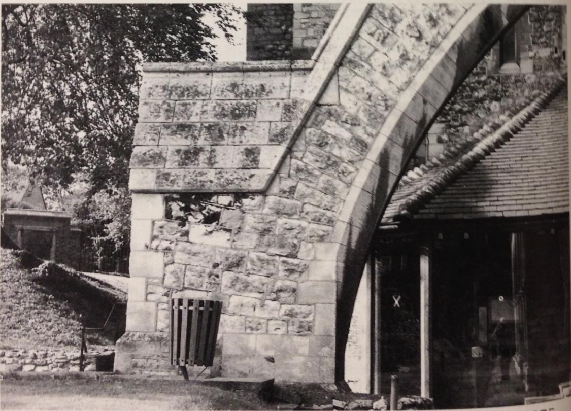
Plate II. Flying buttress to wall of south choir aisle, by Gilbert Scott, 1875. Kenish Rag with dressings of Chilmark stone.
