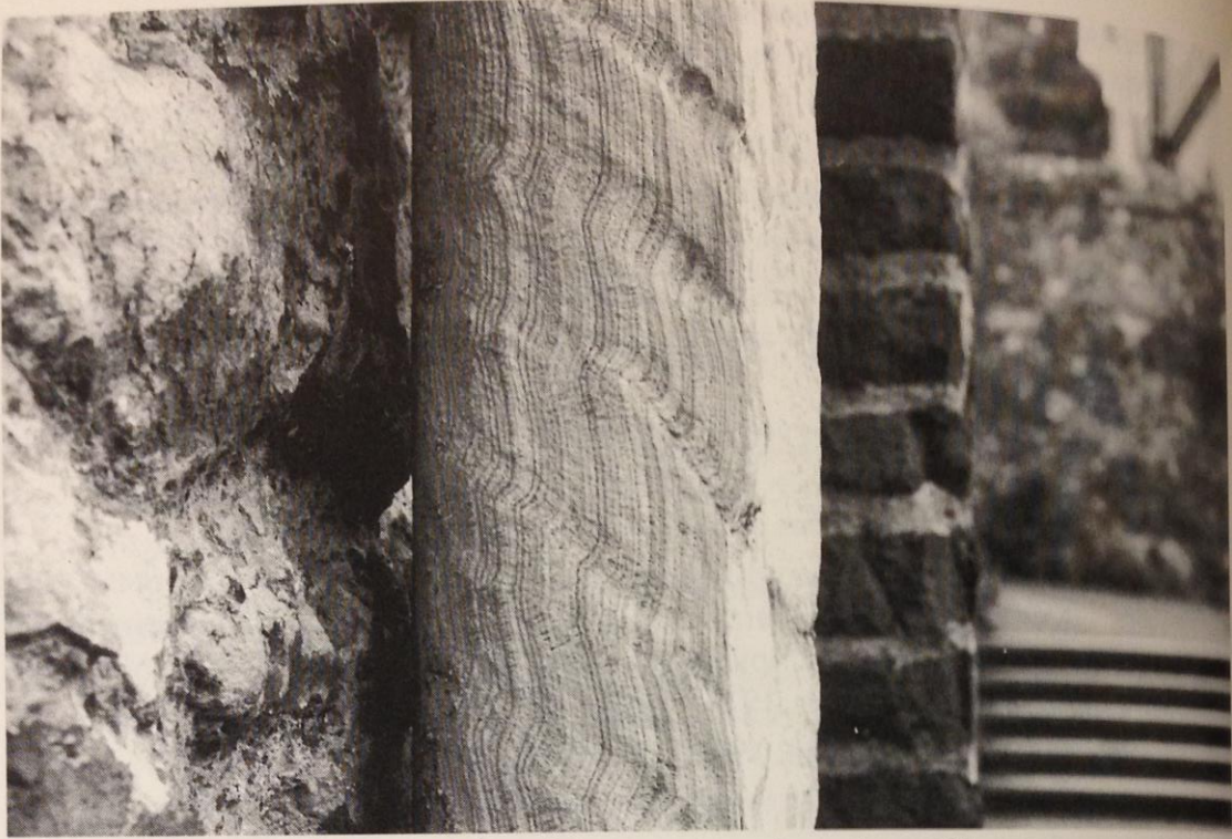
Plate I. In the east range of the cloister, a weathered twelfth-century column of onyx marble, showing undulate bedding.
