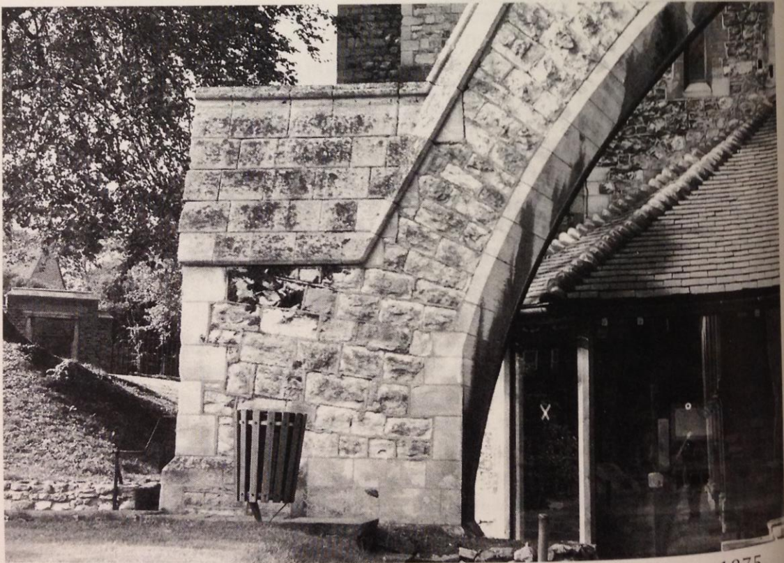
Plate II. Flying buttress to wall of south choir aisle, by Gilbert Scott, 1875. Kenish Rag with dressings of Chilmark stone.
